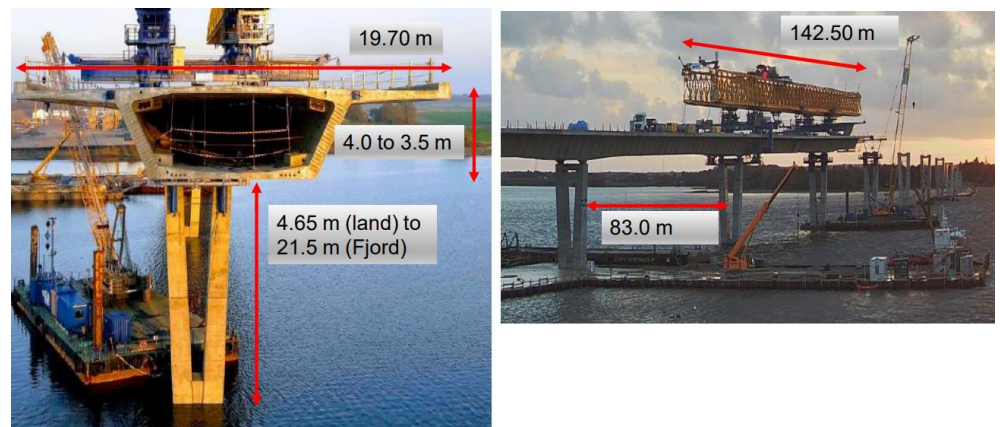
Figur 11 Kronprinsse Marys Bro, precast segmental.
